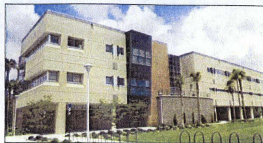
Top: Engineering Building III (Tampa) is the newest of the College of Engineering's seven facilities. The building houses four departments, faculty offices, and state-of-the-art research labs.
